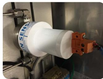
Fig. 2, oxygen sensor
